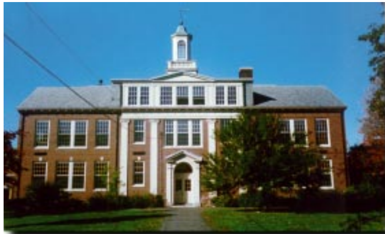
View of Georgian Building
