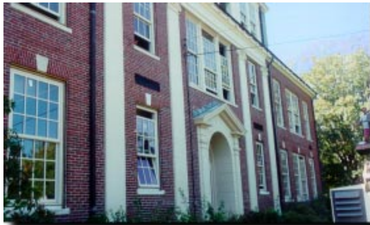
Detail of Georgian Building
