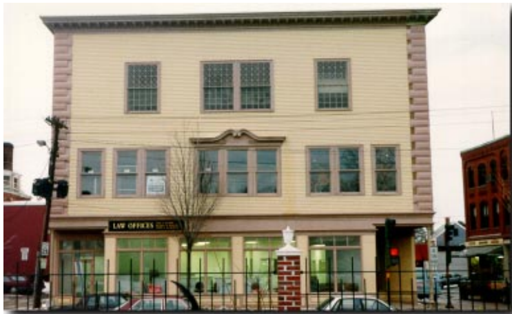
View of Exterior Renovations
