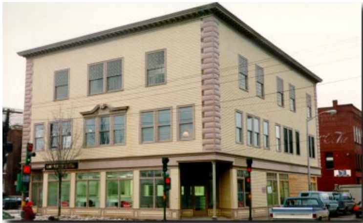
View of Exterior Renovations
