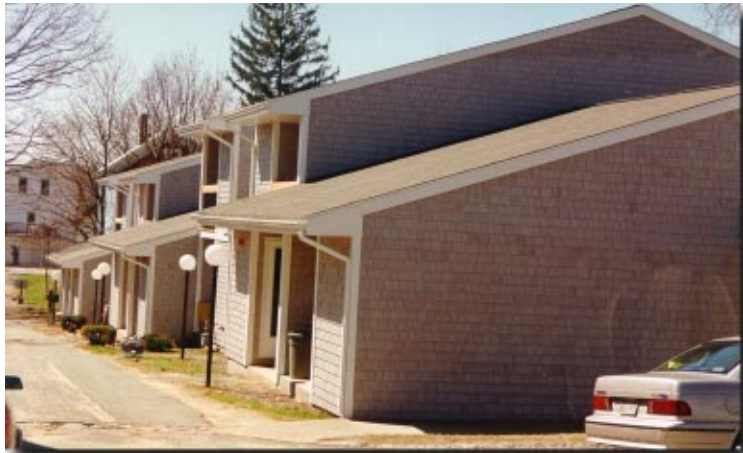
View of Exterior Renovations
