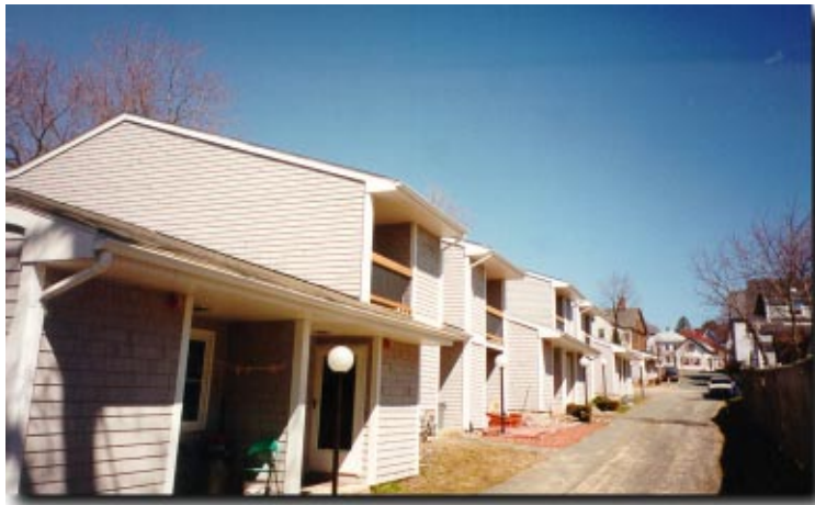
View of Exterior Renovations
