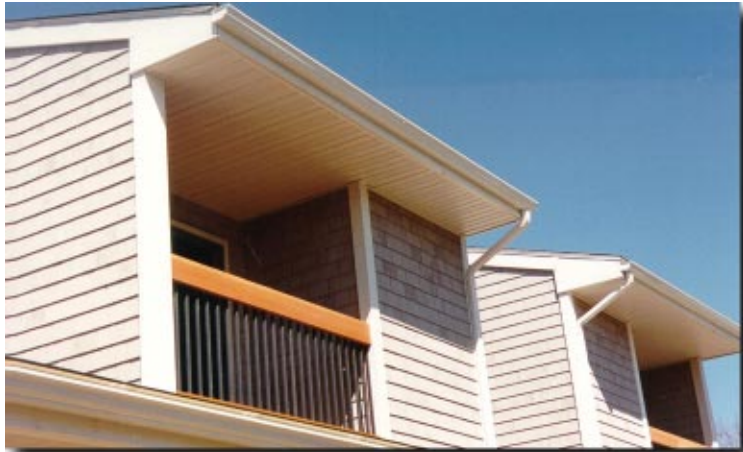
View of Exterior Renovations
